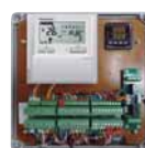
PCB, Power trans, Terminal block
